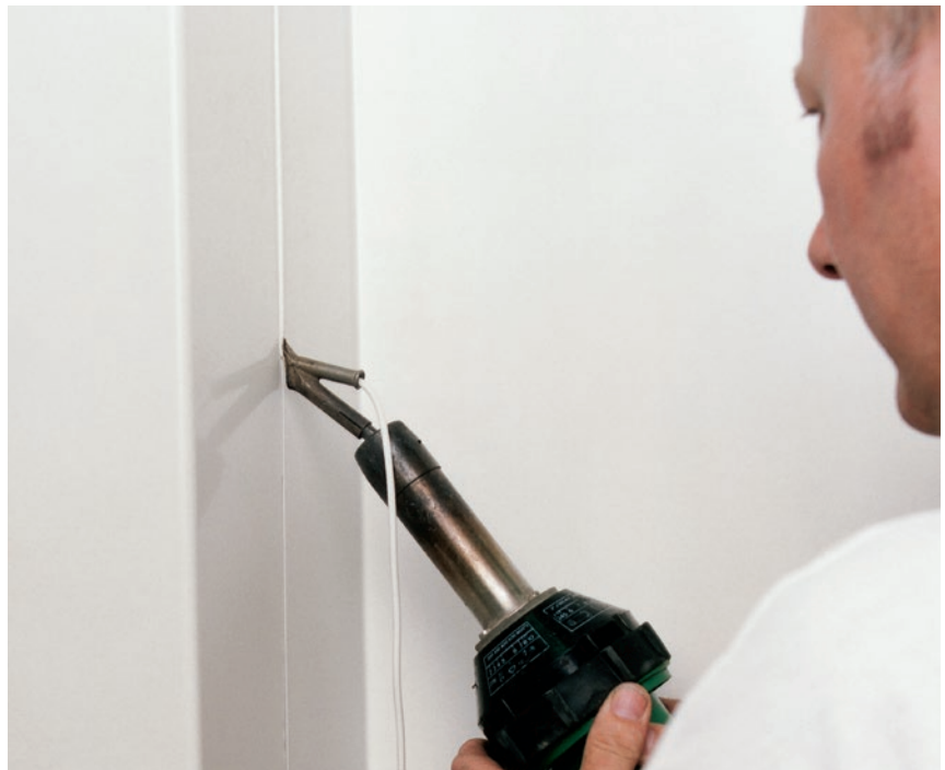
Heat welded installation
